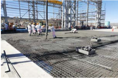
Heavy, labor-intensive traditional reinforcement
